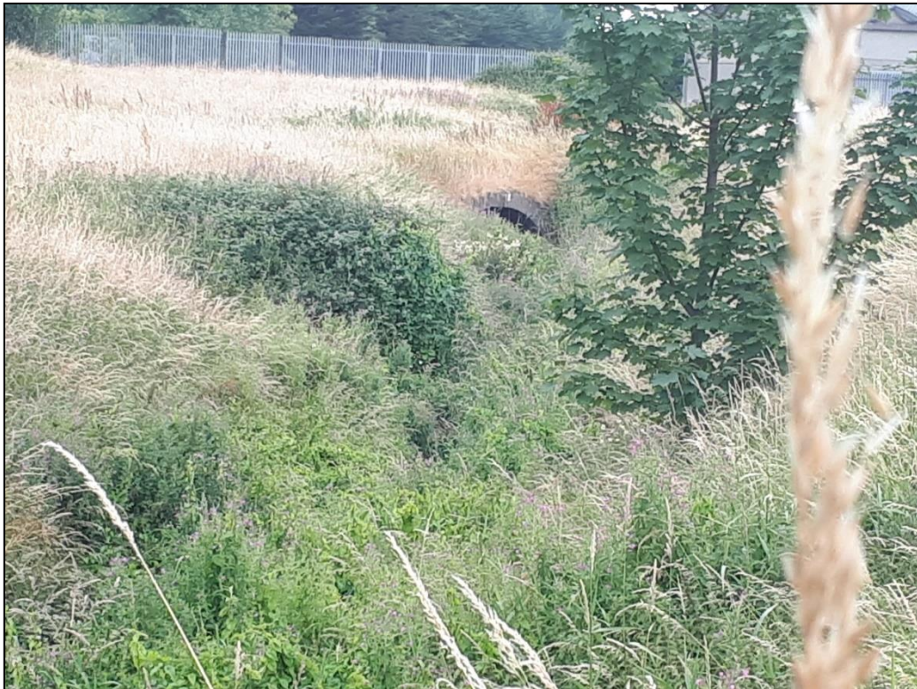
PLATE 14-3 LOOKING WEST AT THE SANTRY RIVER AND CUT STONE SINGLE ARCH BRIDGE
