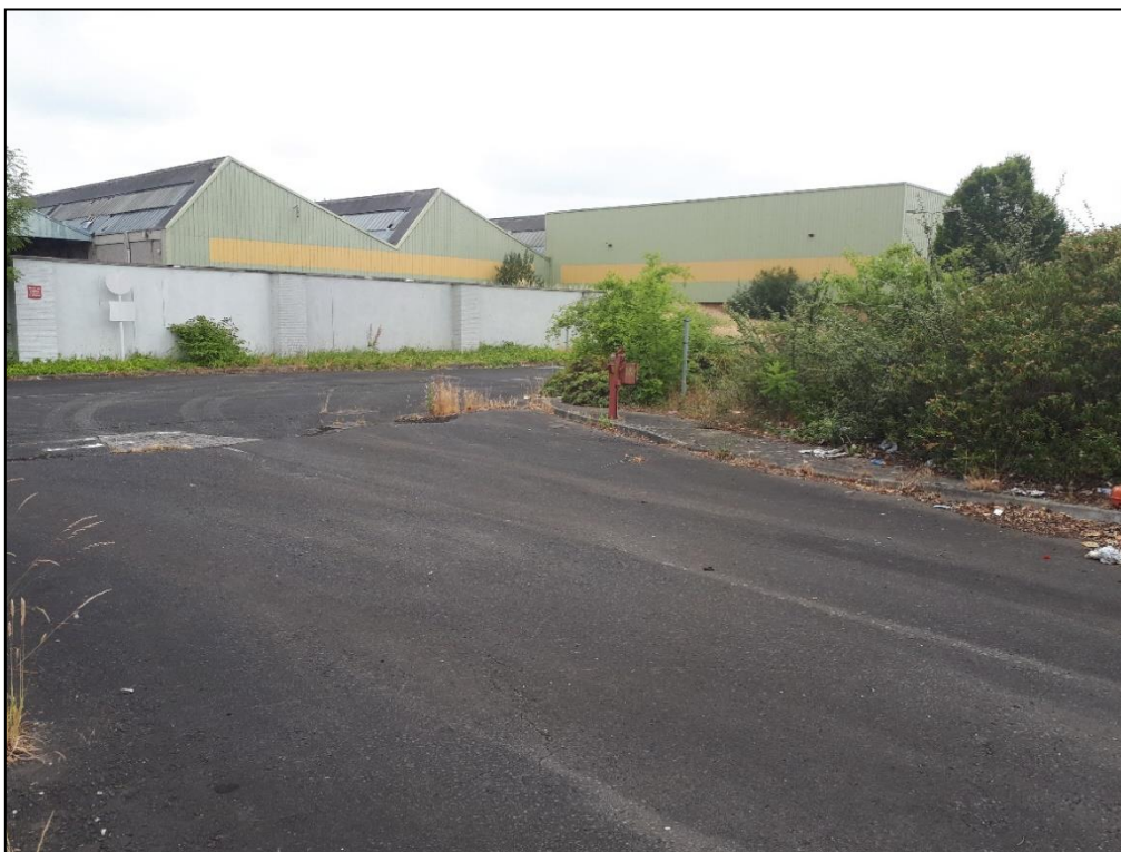
PLATE 14-1 LOOKING SOUTHEAST AT EXISTING FACTORY BUILDINGS AT THE SUBJECT SITE.
